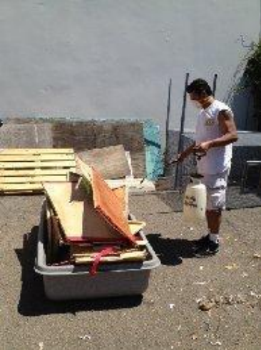
3) Pieces sprayed with Permethrin product
